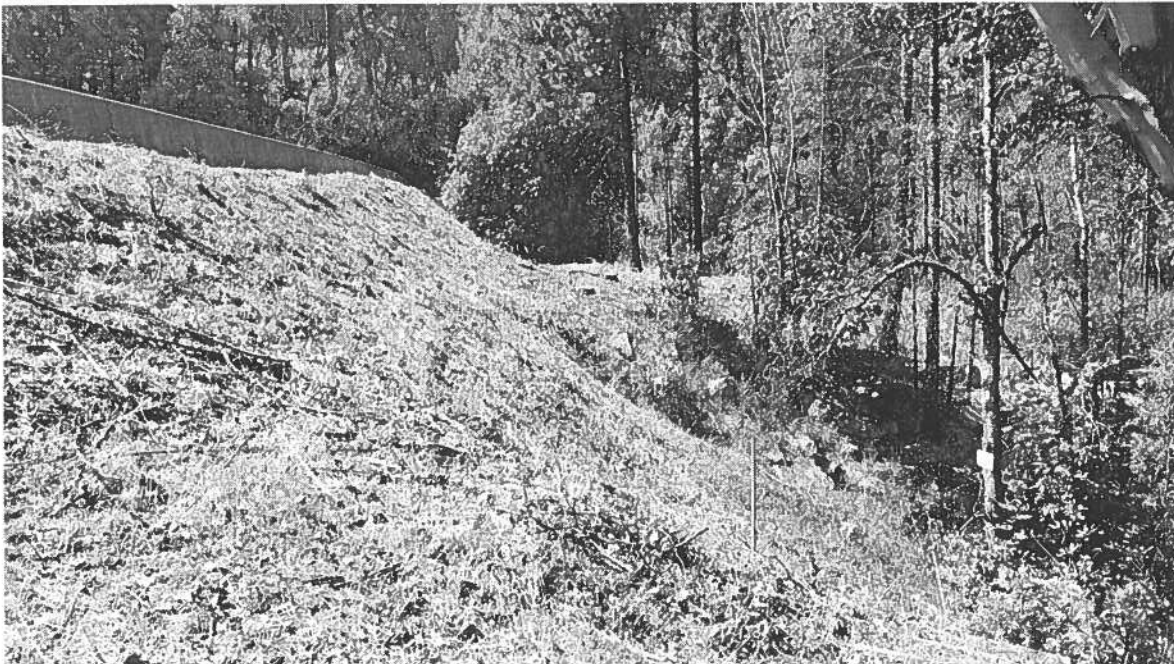
Photo 2: Partial view of the downstream slope toward the left; vegetation control appeared good throughout the dam.
